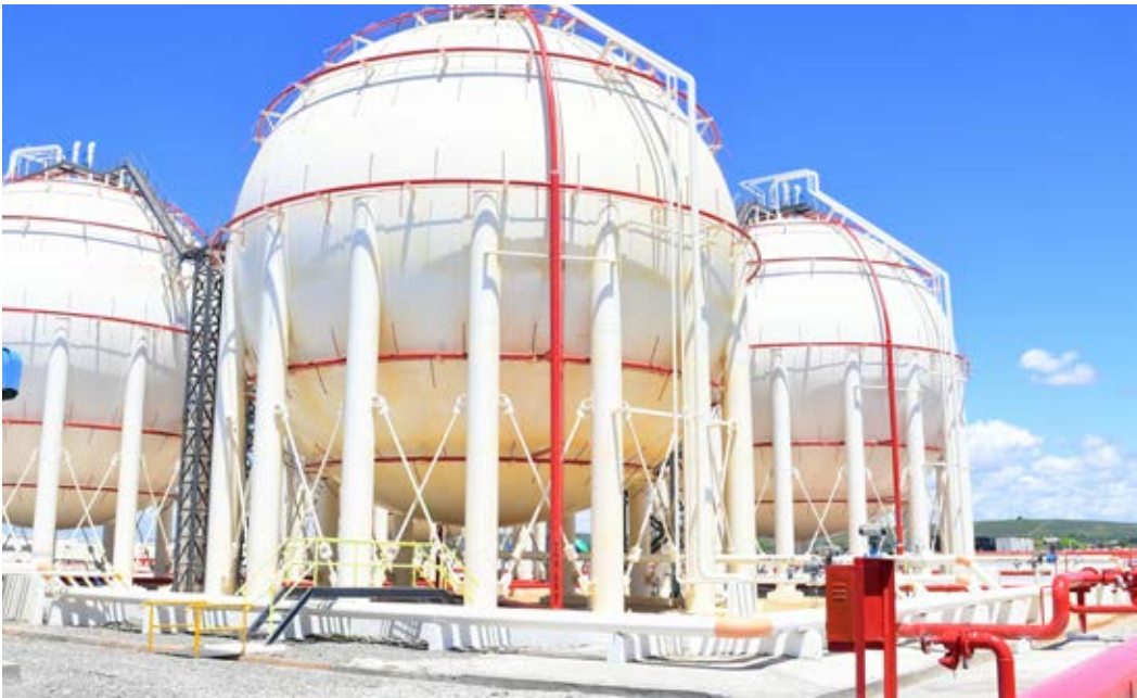
Liquefied Petroleum Gas (LPG) storage tanks at Lake Gas LPG firm in Vipingo, Kilifi.
