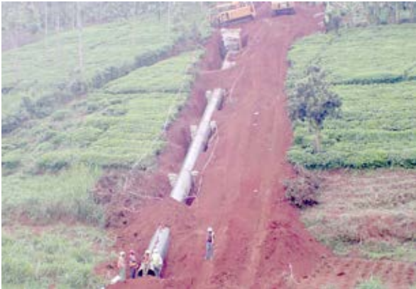
Installation of new water line from Ndakaini to Kirogo water treatment area going on.
